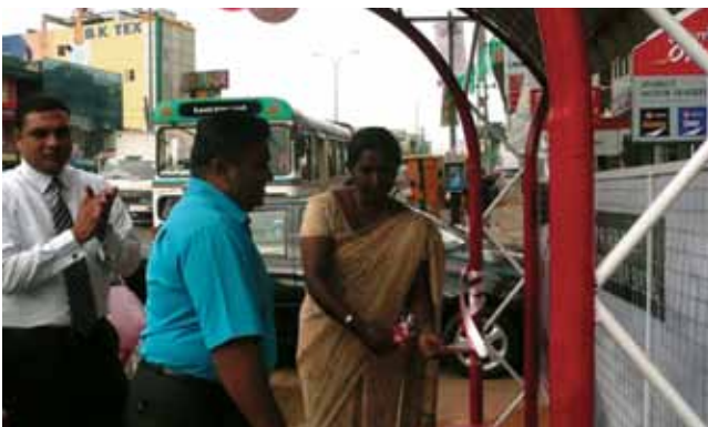
Rebuilding the bus shelter opposite the Kadawatha Branch
