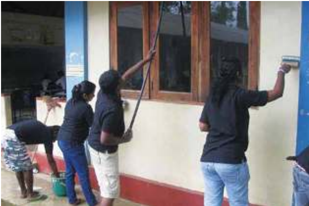
Colour washing of Millaththawa School buildings by the staff of Pan Asia Bank
